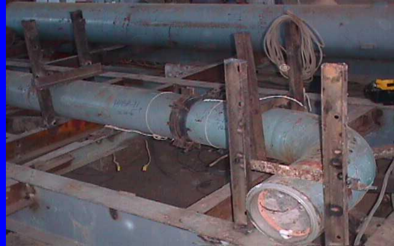
JOINT FITUP COMPLETED AND READY FOR INSPECTION
