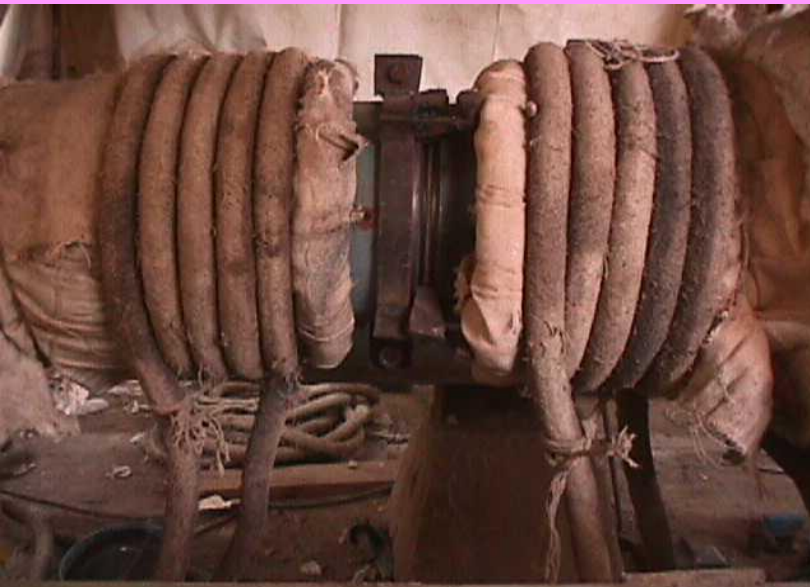
JOINT WRAPPED WITH ANNEALING CABLE ON CERAMIC CLOTH COVERING WOOL INSULATION
