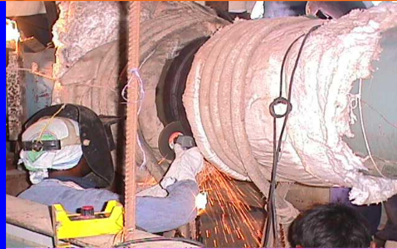
INTER PASS CLEANING DURING SMAW
