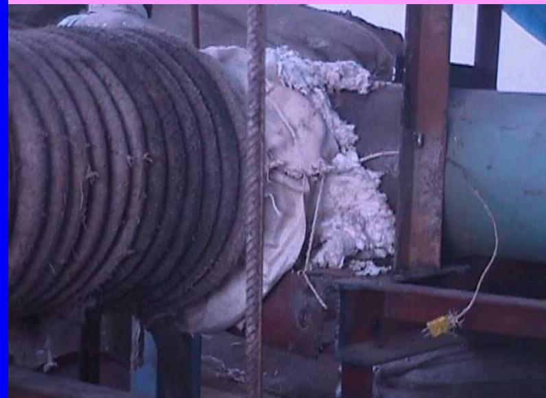
ARRANGEMENT OF ANNEALING CABLE FOR PWHT
