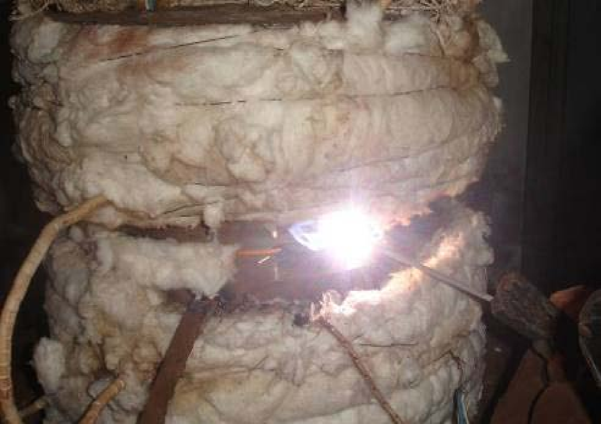
Pre heating & welding arrangement in P 91 steel
