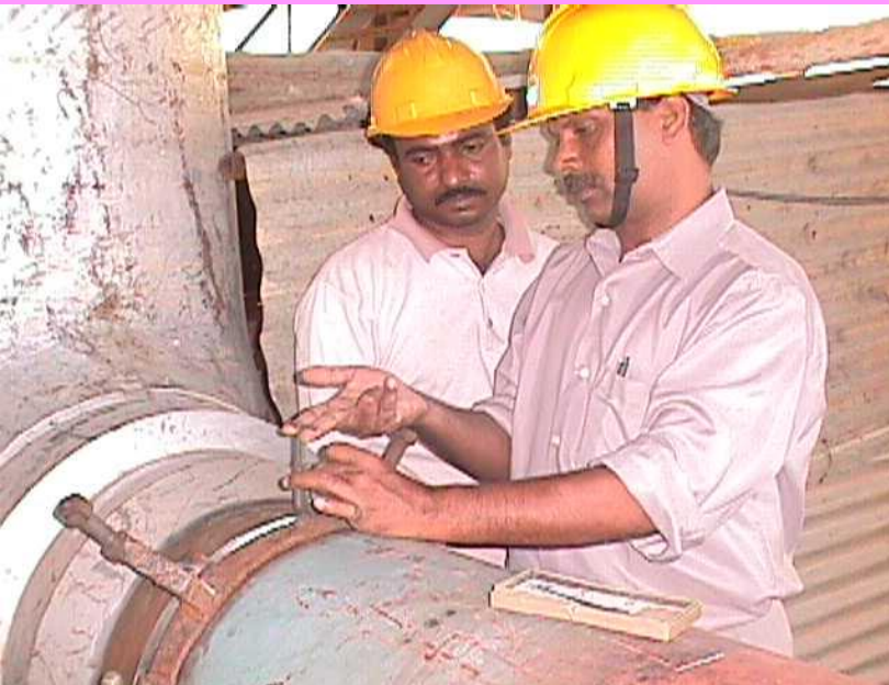
ID MISMATCH CHECKED USING HI-LOW GAUGE
