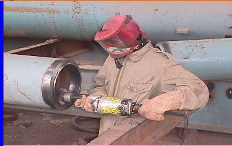
CLEANING OF PIPE ENDS WITH BUFFING WHEEL
