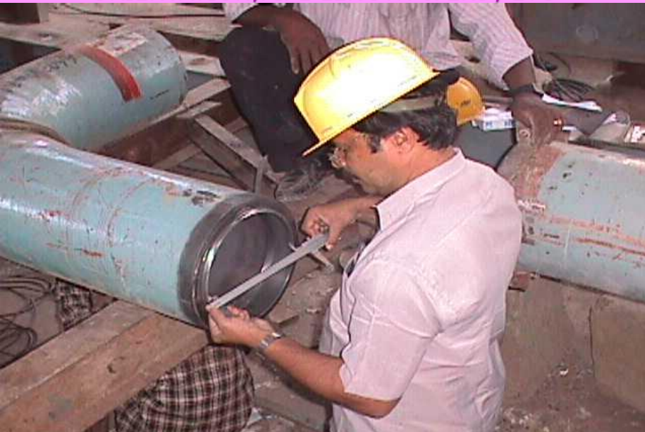
MEASUREMENT OF PIPE ID
