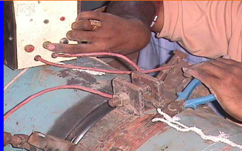
THERMOCOUPLE WELDING ON PIPE
