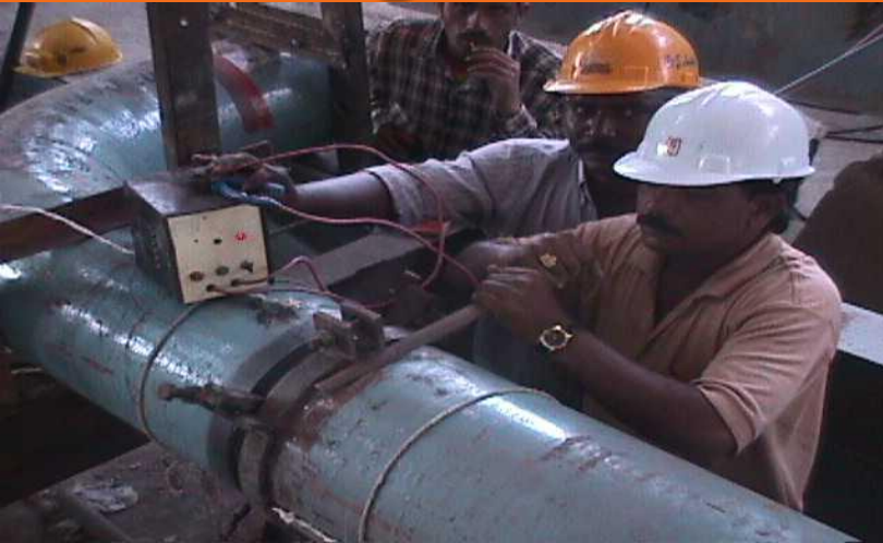
SURFACE PREPARED FOR THERMOCOUPLE WELDING ON PIPE BY FILING
