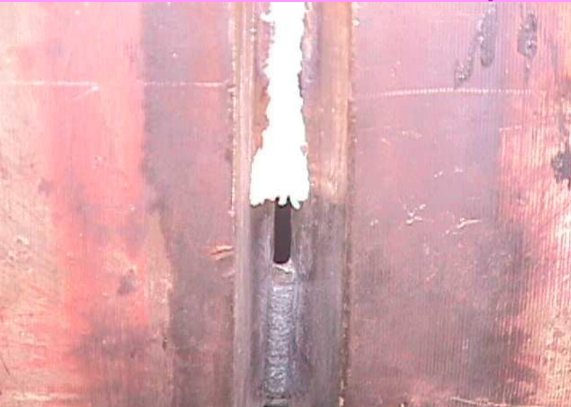
VISUALLY INSPECT ROOT WELDING THROUGH WINDOW OPENING PROVIDED AT BOTH SIDES OPPOSITELY.
