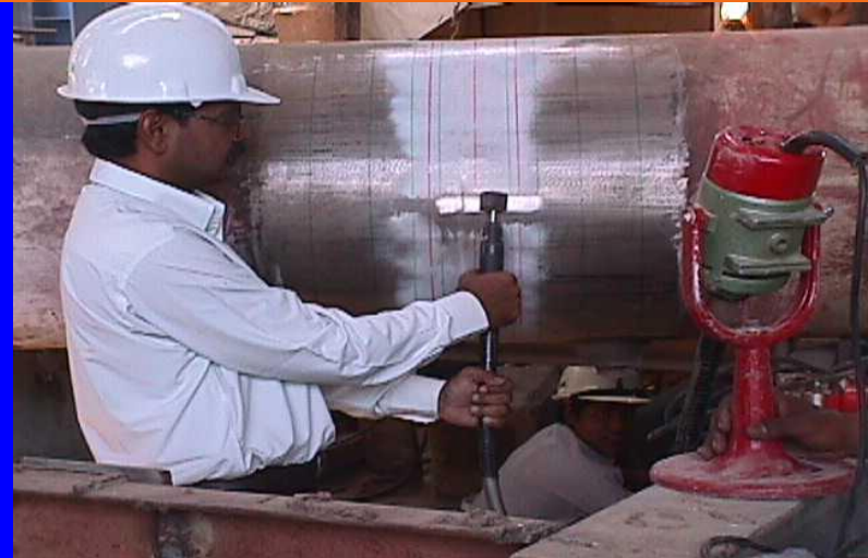
METAL POLISHING AT 3, 6, 9 & 12 O' CLOCK POSITIONS
