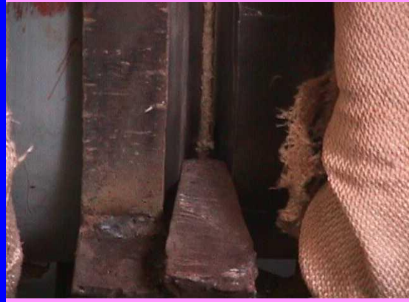
JOINT ROOT GAP CHECKED USING TAPER GAUGE
