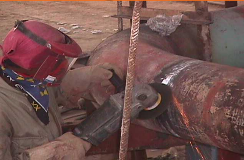
WELD SURFACE FLUSH GROUND FOR NDE
